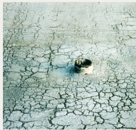
□ Cracked coating
