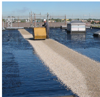
□ Gravel being applied over WeatherScreen
