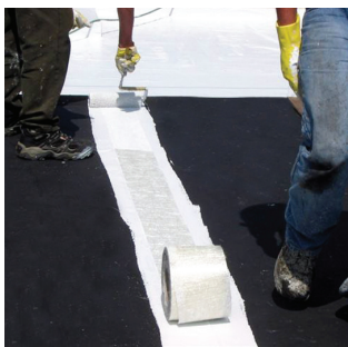
Single-Ply with White-Knight/ White-Stallion reinforcing the seams
