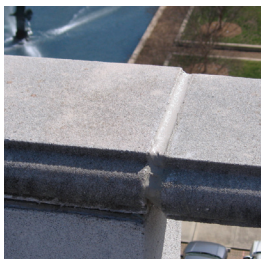
□ Coping Stone sealed with Tuff-Stuff
