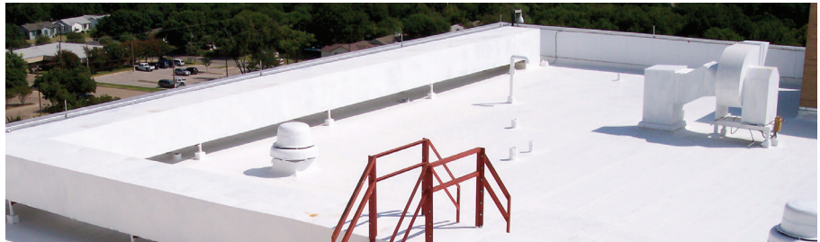
□ After - StressPly SA coated with White-Knight/White-Stallion Plus
