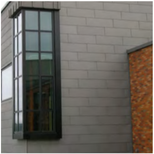
Rainscreens Insulated Wall Panel System will prevent moisture intrusion into your building.
