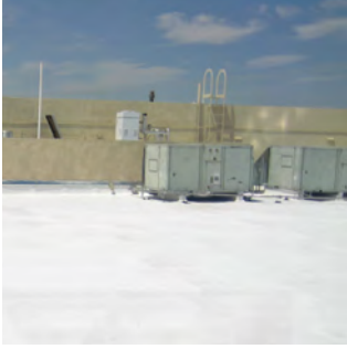
Pyramic® Reflective Coating reduces your buildings heat gain.
